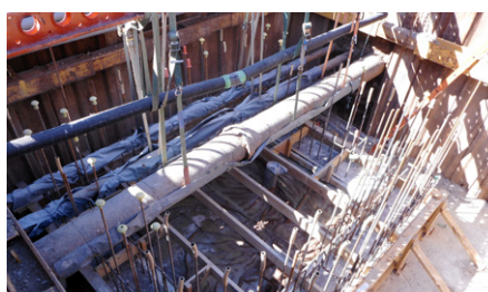
Site enabling works are set to be completed by March 2020.
