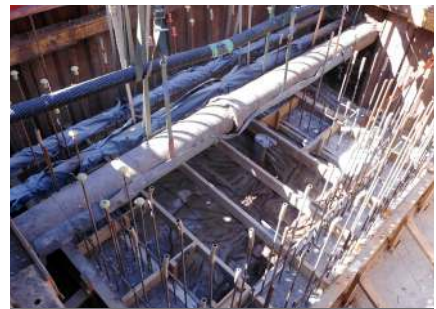
Site enabling works are set to be completed by March 2020.
