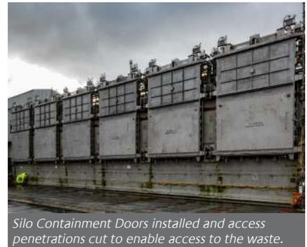
Silo Containment Doors installed and access penetrations cut to enable access to the waste.
